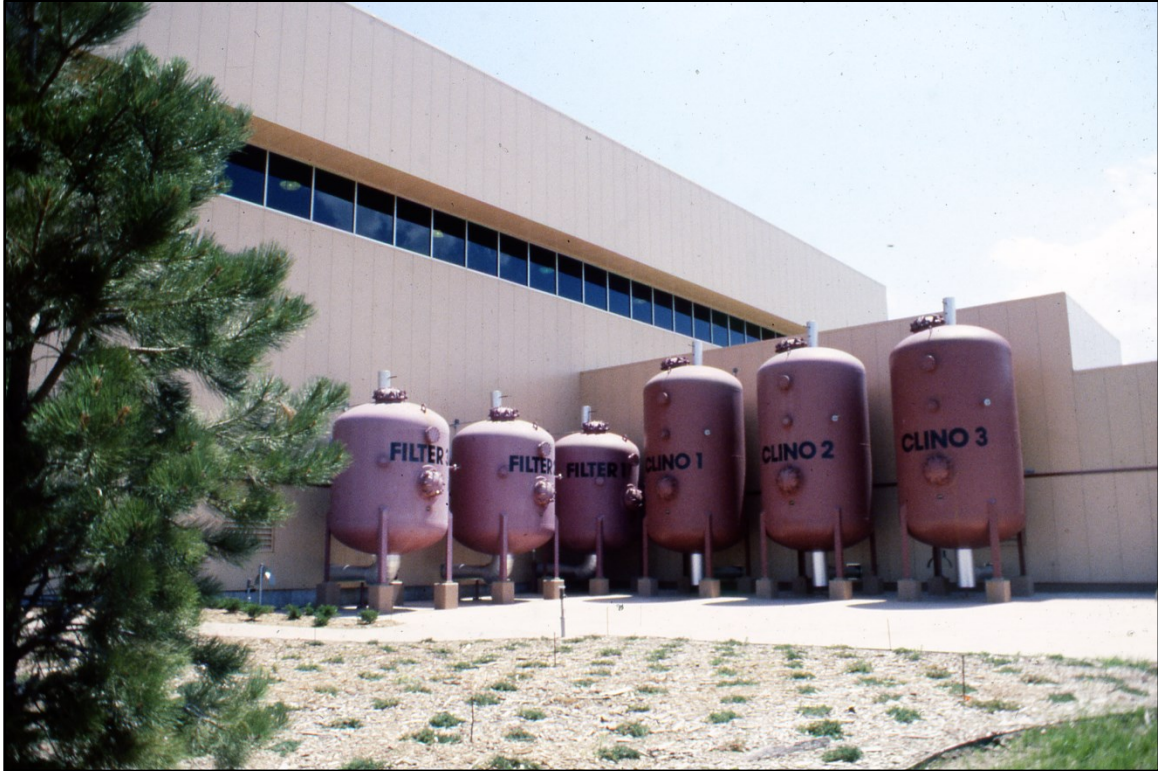
Filter and Clino (Ion Exchange) Tanks Outside Main Process Building
