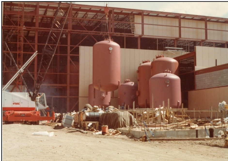
Filter Tank Installation During Construction
